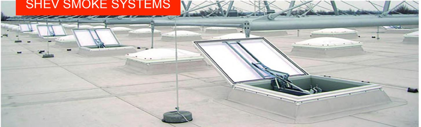
For the essential flow of smoke and hot air out of a building in the event of fire – certified to EN12101-2
